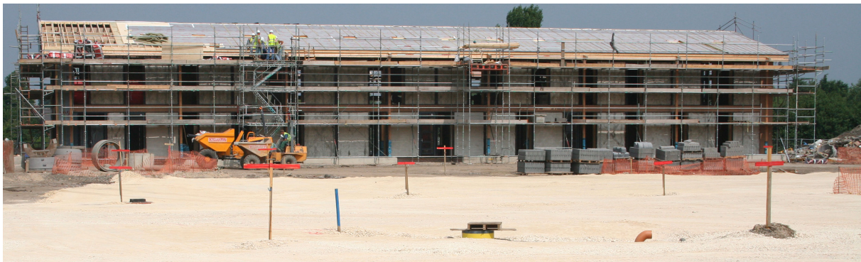
Work on York's Eco-depot October 2006 © Christian Vassie
